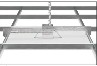
Inspect fixture to ensure arms are resting on the the top of T-Grid and fixture's flanges are fully covering the hole cut in the tile.
