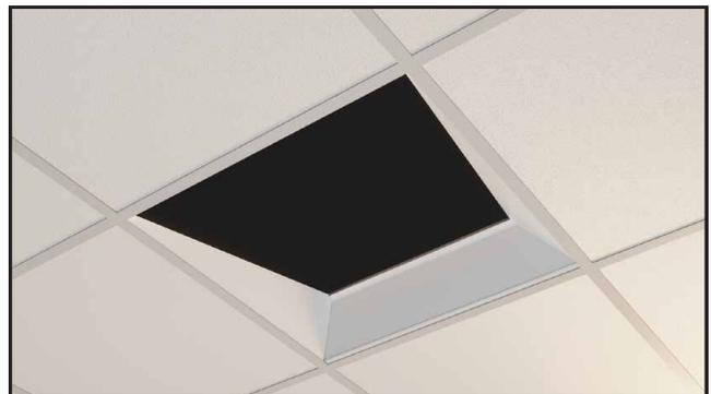
**2** Drop the Loft fixture into the T Grid in correct orientation.
