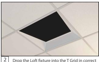
Drop the Loft fixture into the T Grid in correct orientation.
