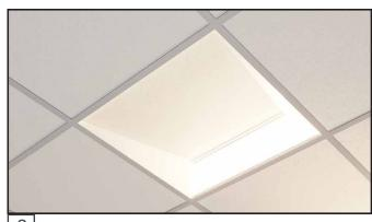
Place the ceiling tile on the top of the fixture to complete installation.
