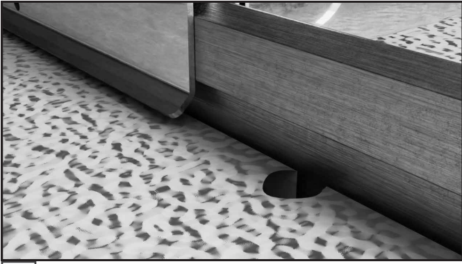
3 Create a small notch in the ceiling tile for wiring to pass through.
