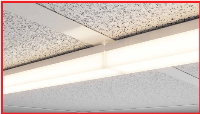
1 Once the first section of the fixture is installed, hold the second section up to the ceiling and align it with the the joining tongue.
