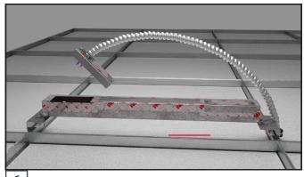
Attach BX power supply to driver using necessary connections, then attach access plate to driver.
