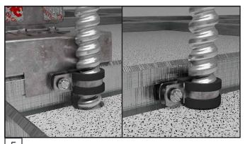
Secure loop clamp to either the designated hole one the driver box clip or into the T-Grid.
