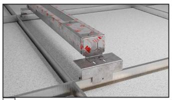
Install remote driver box as close as possible to the wire passthrough hole by clipping it to the top of the T-grid.
