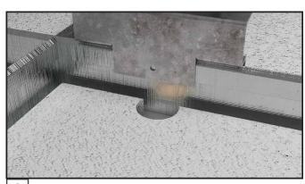
Create a notch in the ceiling tile for 1/2" conduit to pass through.
