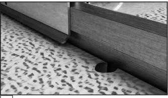
Create a small notch in the ceiling tile for wiring to pass through.
