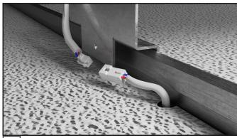
6 Connect low voltage power from fixture to driver wires using provided connectors. Attach safety wire to structure.
