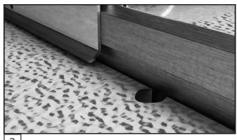
Create a small notch in the ceiling tile for wiring to pass through.
