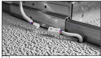
Connect low voltage power from fixture to driver wires using provided connectors.
