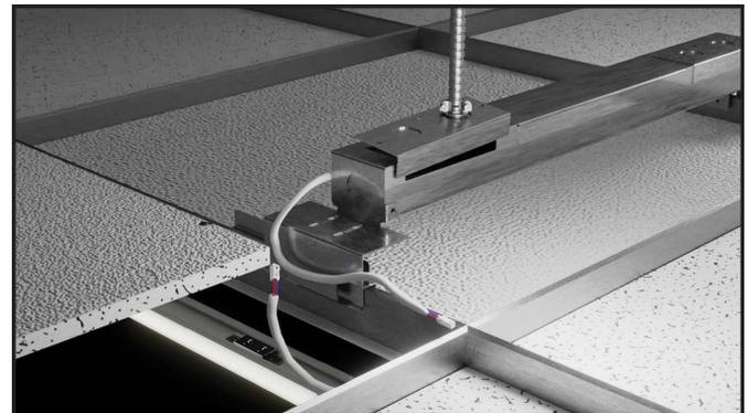
2 Attach BX power supply to driver using necessary connections. Run low voltage wire provided towards fixture. Low voltage wire from driver remains in ceiling.
