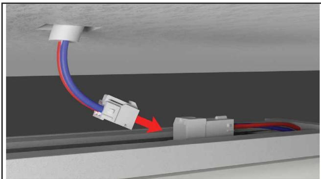
13 Attach the power cable from the fixture to the supplied driver housing.
