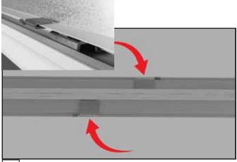
Push fixture up against T-Grid and roate clips until they are parallel with the fixture and fully engaged with T-Bar.
