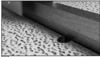
6 Create a small notch in the ceiling tile for wiring to pass through.
