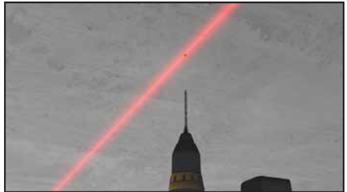
2 Drill holes using 3/16 drill bit at least 1 1/2" in line at the distances specified for that fixture length in the cut sheet/shop drawings.
