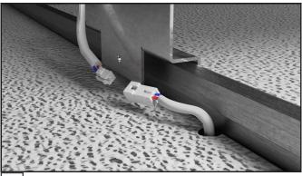
7 Connect low voltage power from fixture to driver wires using provided connectors.
