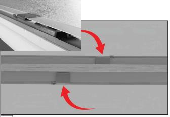
Push fixture up against T-Grid and rotate clips until they are parallel with the fixture and fully engaged with T-Bar.
