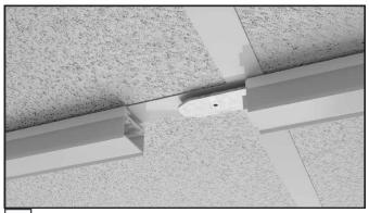
Once the first section of the fixture is installed, hold the second section up to the ceiling and align it with the the joining tongue.
