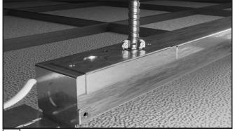
Attach BX power supply to driver using necessary connections. Run low voltage wire provided towards fixture. Low voltage wire from driver remains in ceiling.
