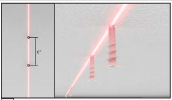
Install included Drywall Anchors on the line at the distances specified for that fixture length in shop drawings.
