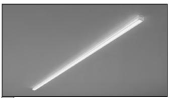
Turn power on to fixture to ensure it is connected properly, then close up driver box hole.
