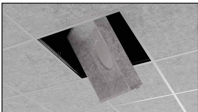
1 Install fixture into ceiling grid.
