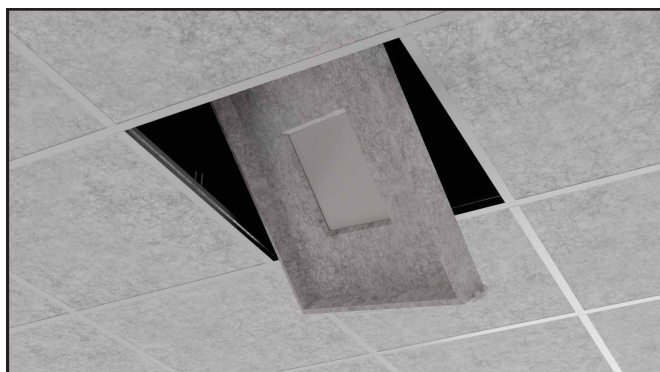
1 Install fixture into ceiling grid.
